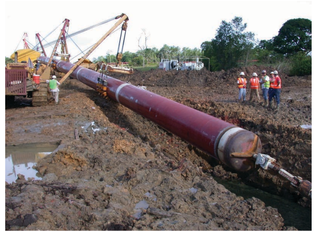
A 56-inch gas pipeline in Trinidad.
