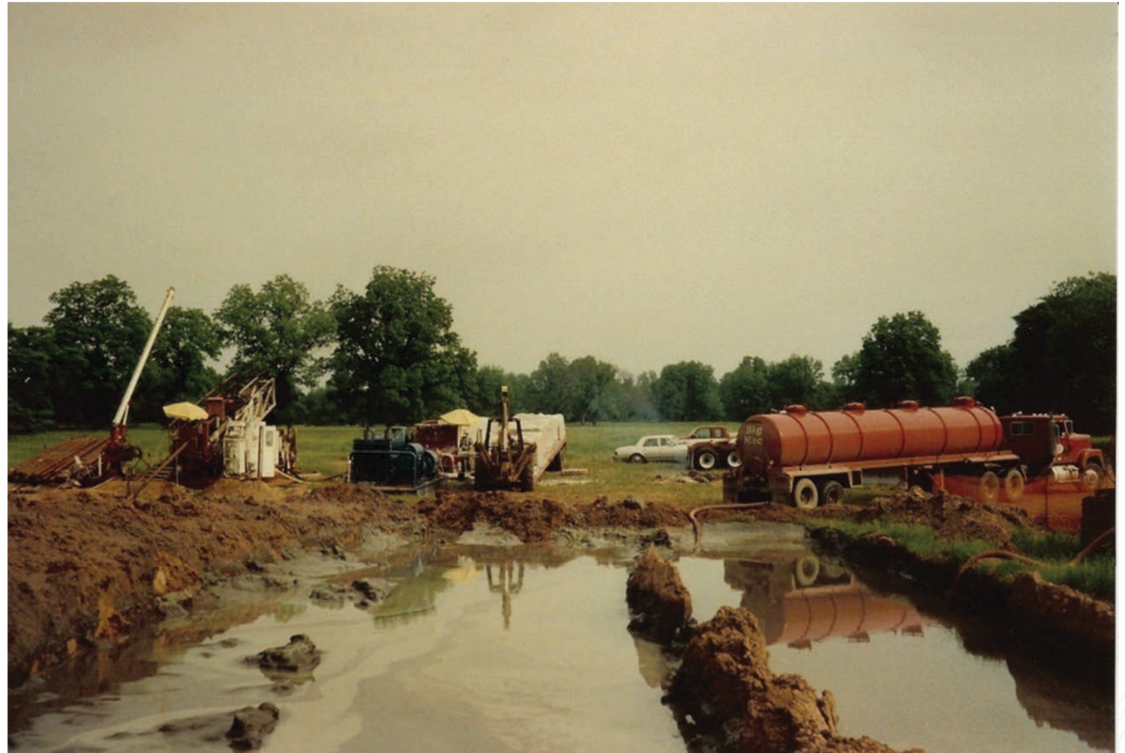
Drilling fluid and cuttings contained in large open pits.
