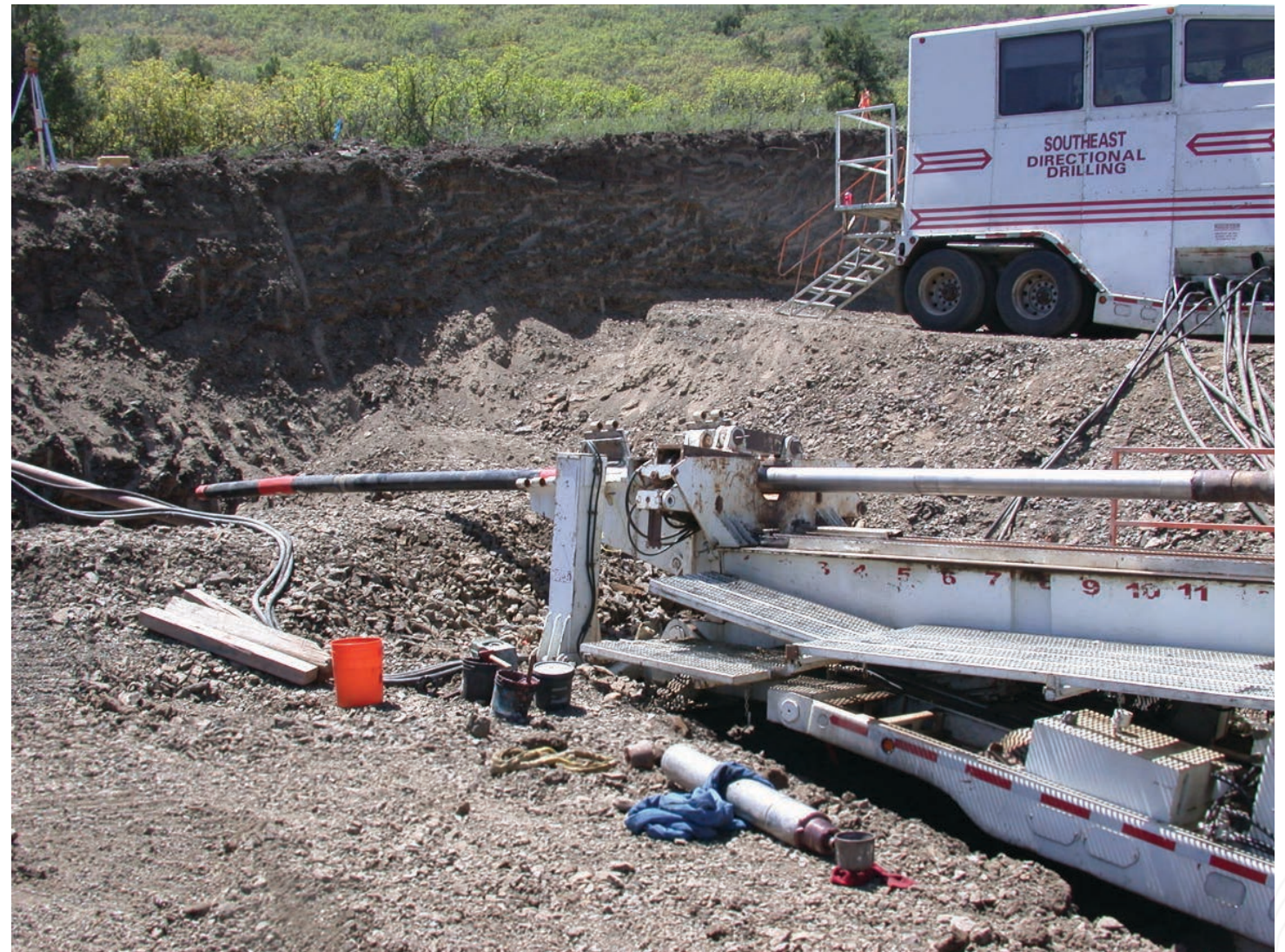
A Bottom Hole Assembly with a positive displacement mud motor.
