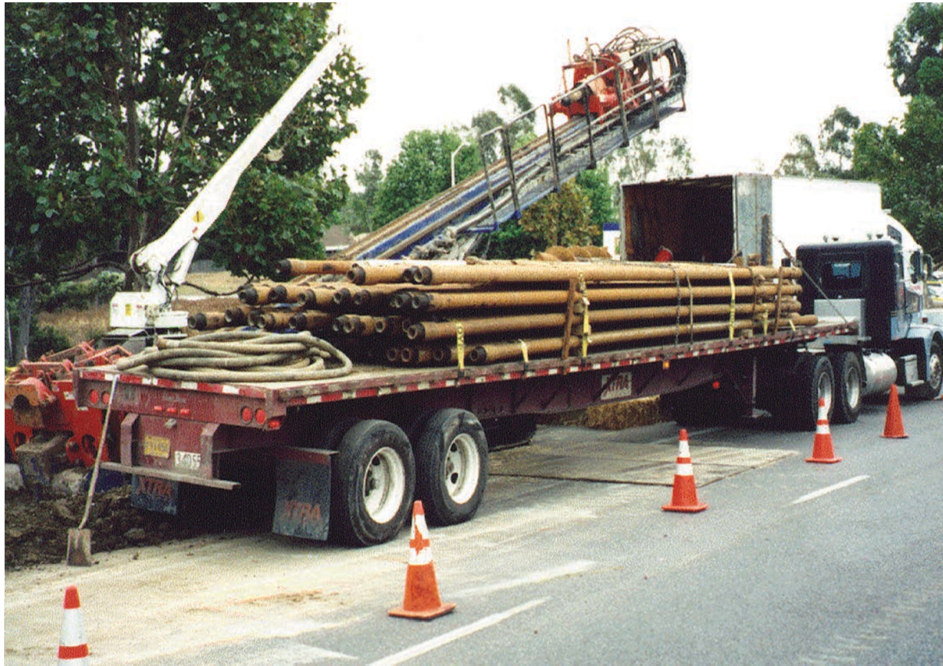
Joints of Range 2 drill pipes (~31 feet long)
