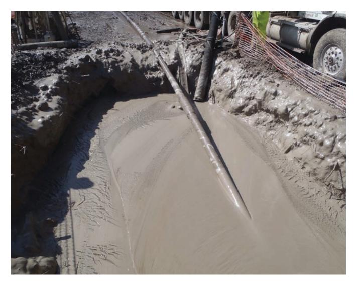
HDD drilling fluids are the elixir between the soil formation and the deployed downhole tools. Drilling fluid is a mixture of bentonite clay and water. Sometimes other additives are mixed in. It's function is to:
