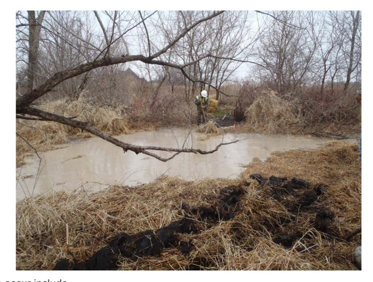
locations where drilling fluid surface releases can occur include exploratory boring locations, or along the edges of existing subsurface structures such as basements, piles or utility poles.
