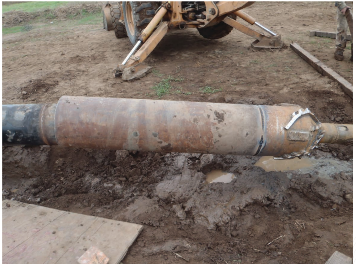
A gravel shield welded to the pullback assembly to cover the swivel and pullhead.
