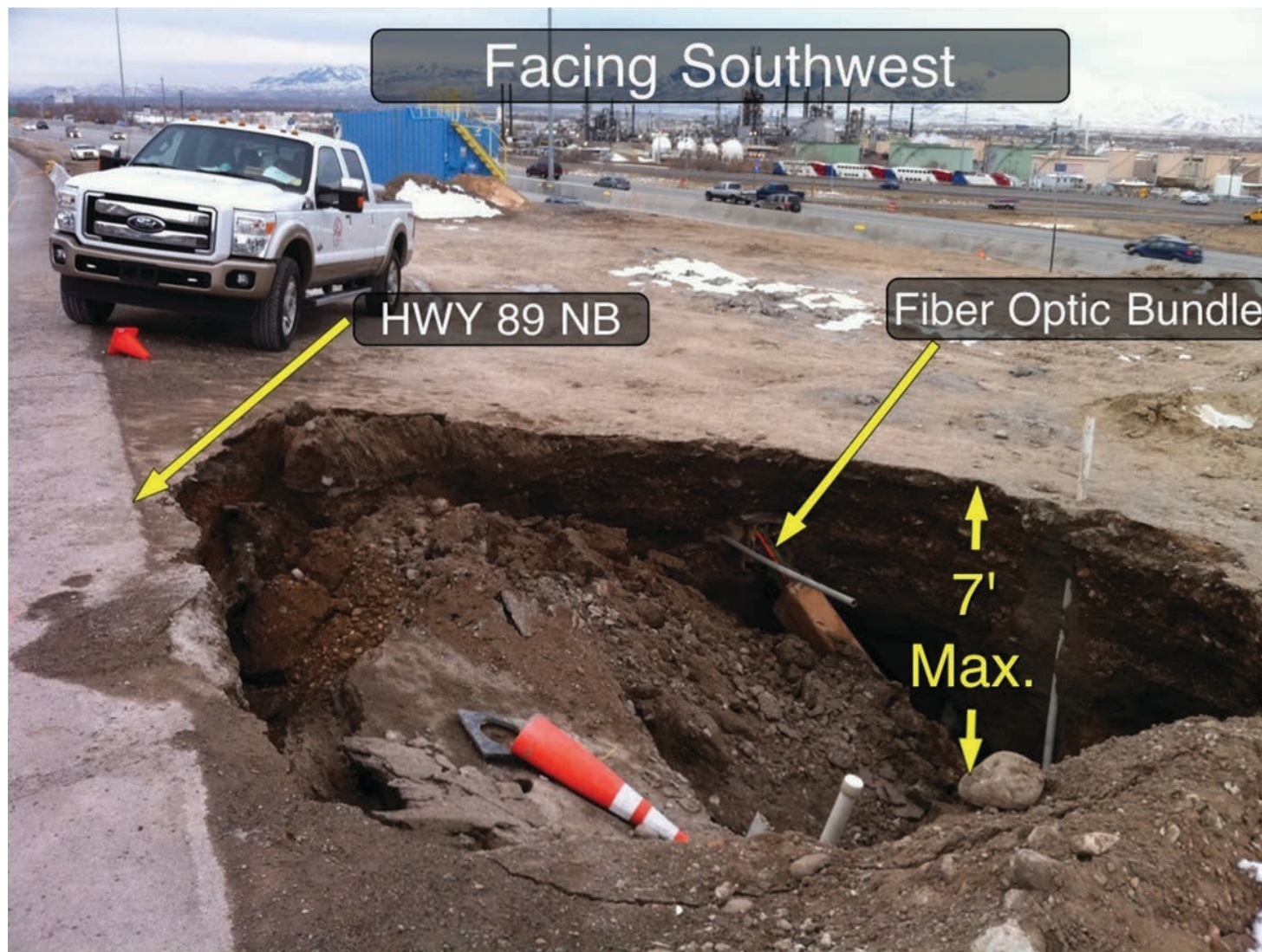
A sinkhole that formed along an HDD alignment as a result of hole instability through a dry hole section in granular soils.
