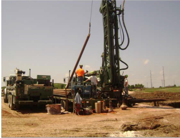
FIGURE 2.1- DRILLING RIG AND TENDER AT THE JTEC SITE ON MAY 21, 2010
