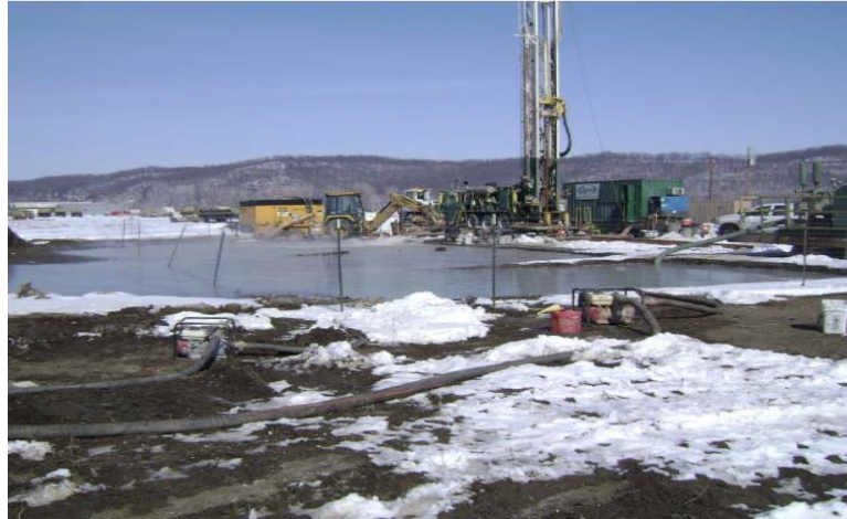
FIGURE 2.6- DRILLING RIG AND CUTTINGS MANAGEMENT AT THE IATAN SITE, MARCH 2, 2013.
