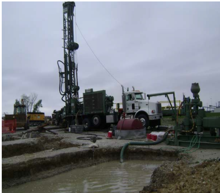
Figure 2.4: Drilling Rig and Mud System at the Thomas Hill site, April 4, 2012.
