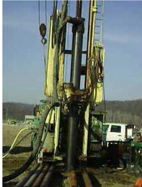
FIGURE 2.5- ADVANCE CASING WHILE DRILLING SYSTEM AT THE IATAN SITE, NOVEMBER 30, 2012
