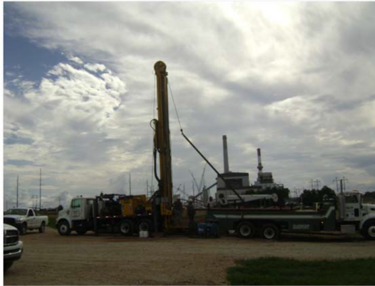
FIGURE 2.2- CORING RIG AND TENDER AT THE JTEC SITE, JULY 6, 2010
