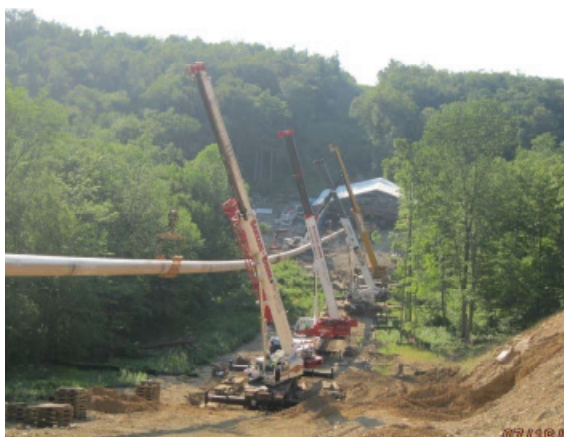
GeoEngineers provided construction consulting services—pipe pullback pictured here—during the challenging 5,800-foot Lake Conway HDD crossing in New Jersey.
