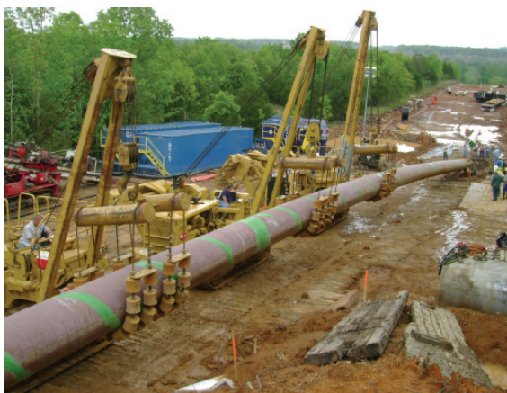
GeoEngineers observed construction of the 36-inch-diameter HDD installation beneath the Little Red River in Arkansas.
