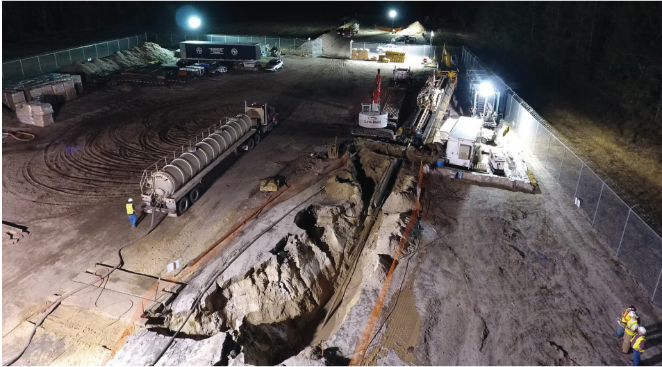
Drilling operations underway in Florida for the 36-inch-diameter, 3,991-foot-long Suwannee River HDD as part of the Sabal Trail Transmission Pipeline Project. Drilling the pilot hole began December 1, 2016, and pullback was complete January 16, 2017.
